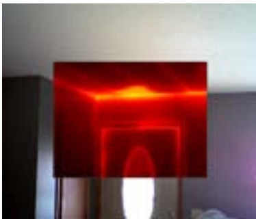
Recessed blown-in attic insulation
